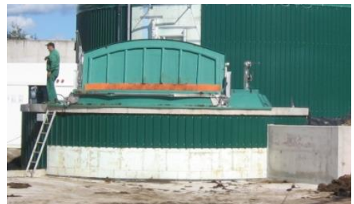
Hydrolysis with closed and open flap for feeding
