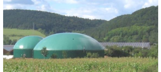
Digester, digestate storage and solar panels
