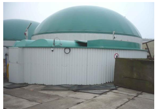
Hydrolysis In the foreground: flap for daily feeding
