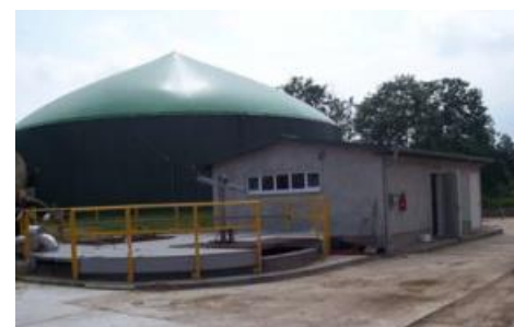
In the foreground: mixing tank In the background: interim storage At the right : operations building
