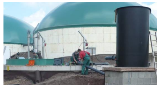
In the foreground: Bio filter In the middle: Hydrolysis In the background: Digester
