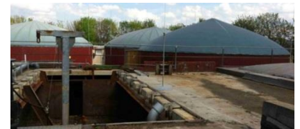
Converting the dry digester to a mixing pit, 2012
