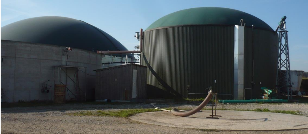
Pre tank, digester and post digester. Aerial photo of the plant before closing of the post digester
